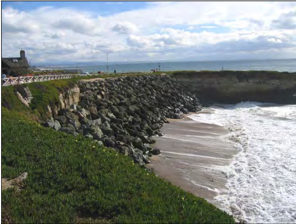
Figure 5: Riprap covering up significant amount of beach area in Santa Cruz, California, near the intersection of Westcliff Drive and San Jose Avenue.
