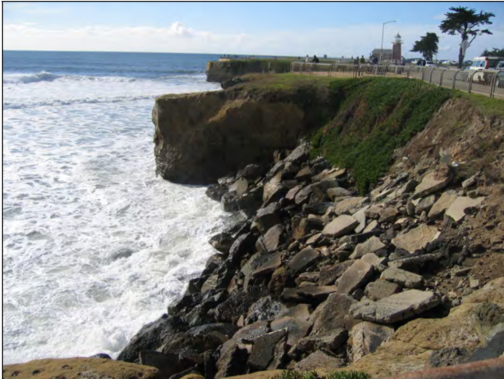
Figure 2: Concrete blocks used as riprap near Lighthouse Point in Santa Cruz, California.
