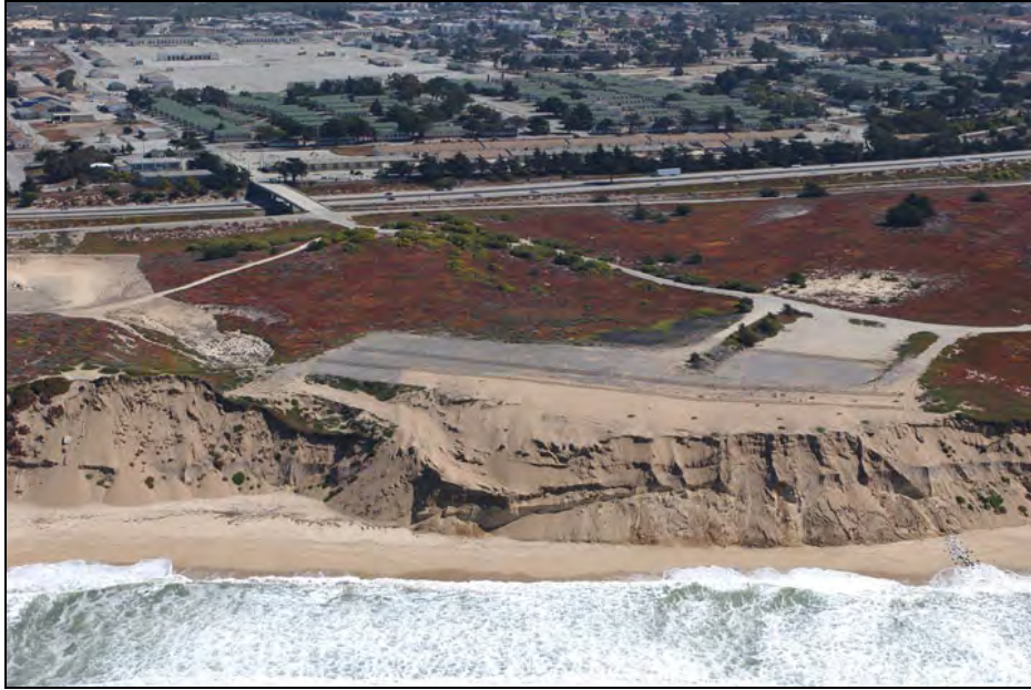
Figure 1b: Oblique aerial photograph of the former Stillwell Hall location after the building and associated coastal protection structures were removed in March 2004. Photograph copyright © 2002 Kenneth & Gabrielle Adelman ( http://www.californiacoastline.org/ ).
