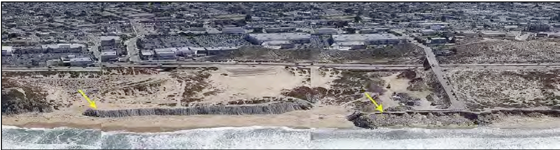
Figure 5.2: Aerial photo mosaic of the concrete slurry “ridge” and other hard structures (indicated with yellow arrows) at the end of Tioga Road in Sand City, California. Photographs taken October 2004; copyright © 2002 Kenneth & Gabrielle Adelman ( http://www.californiacoastline.org ).
