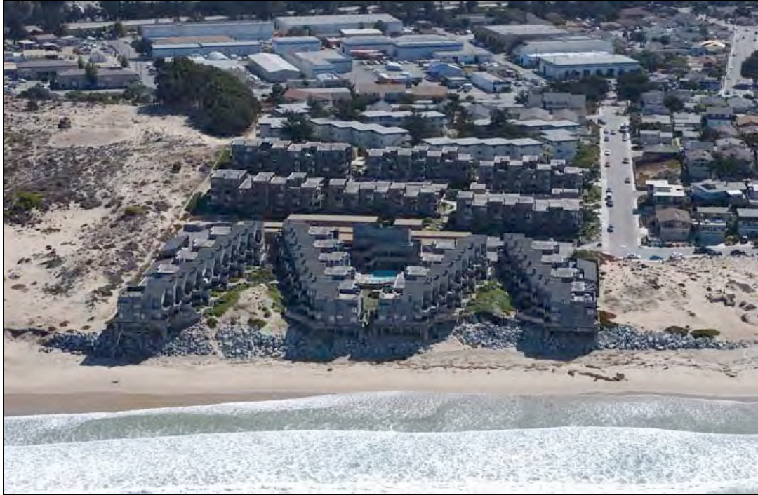
Figure 5.6: Aerial photograph of extensive riprap in front of the Ocean Harbor House Condominiums in Monterey, California. Photograph taken October 2004; copyright © 2002 Kenneth & Gabrielle Adelman ( http://www.californiacoastline.org/ ).
