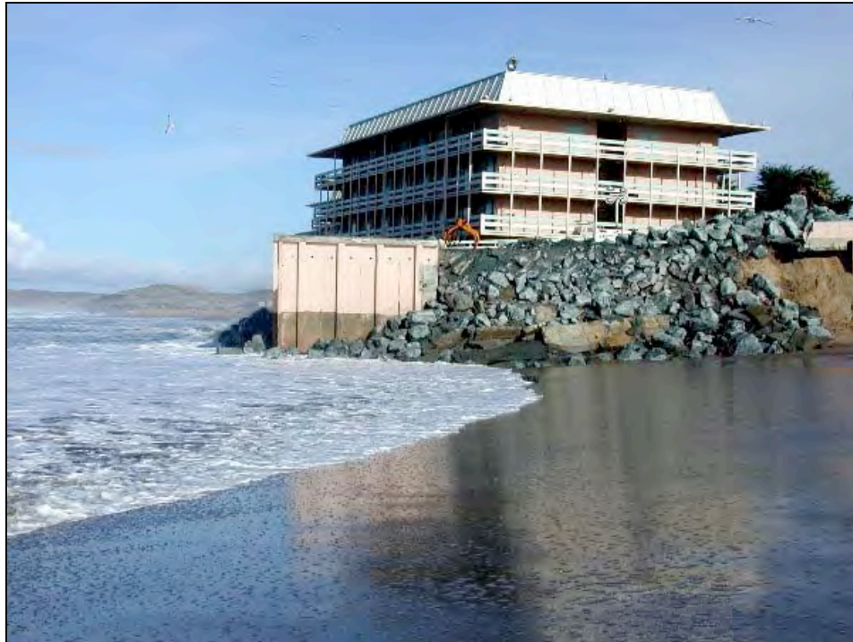
Figure 5.4: Wave run-up against the Monterey Beach Hotel seawall and riprap during the winter of 2002. Lateral access is cut off because of this coastal armoring. Photo: Doug Smith, CSUMB.
