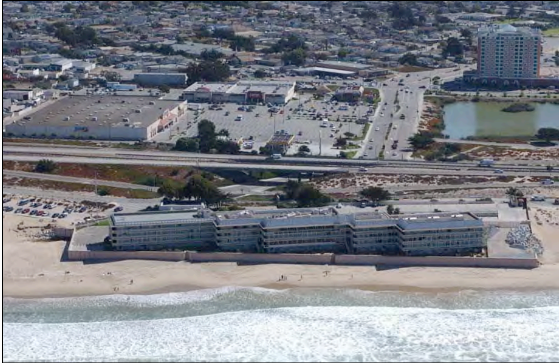
Figure 5.3: Aerial photograph of the seawall and riprap (at the far right end of the seawall) protecting the Best Western Monterey Beach Hotel in Seaside, California. Photograph taken October 2004; copyright © 2002 Kenneth & Gabrielle Adelman ( http://www.californiacoastline.org/ ).
