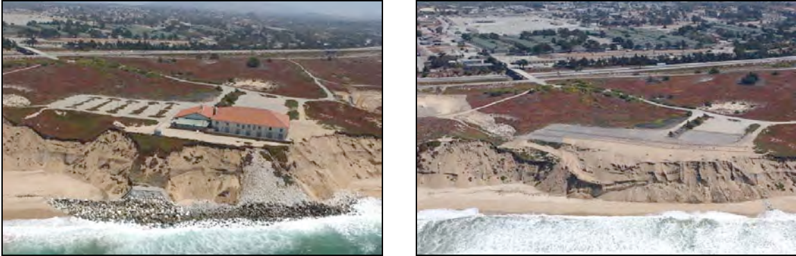
Figure 4.1: The former Fort Ord soldier's club, Stillwell Hall, was demolished in 2004 because attempts to save the structure from collapsing into the ocean by emplacing riprap in front of the dunes proved to be too costly and ineffective. Left photo taken August 2003, prior to demolition. Right photo taken October 2004 after removal of structure and all riprap. Photographs copyright © 2002 Kenneth & Gabrielle Adelman ( http://www.californiacoastline.org/ ). See Figure 5.1 for location.
