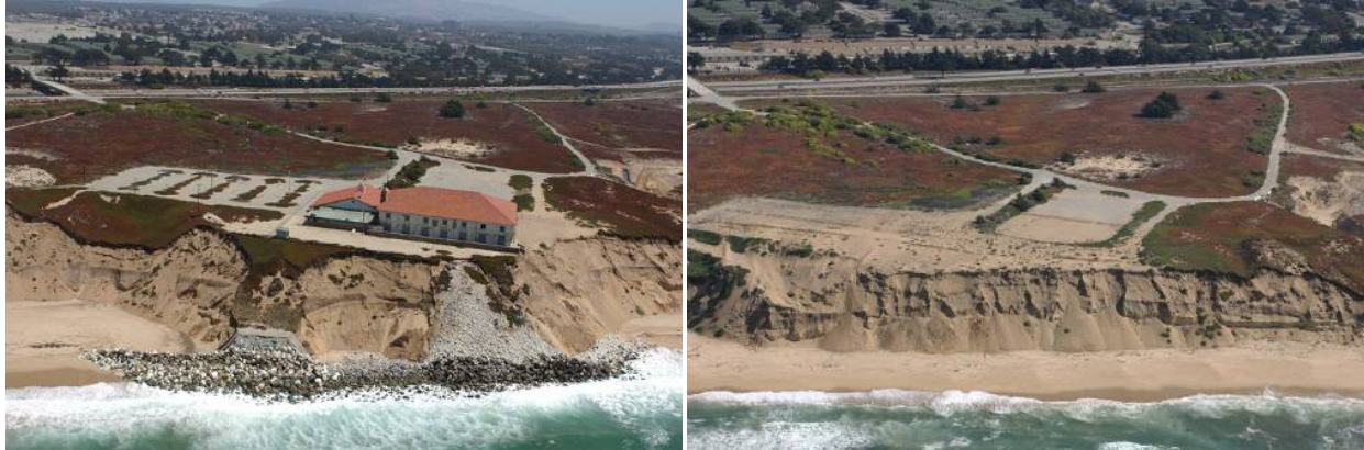
Figure 18 Stillwell Hall on Fort Ord. Photo on left taken in 2002 shows the building and revetment, and photo on right from 2005 shows the site, with recovered beach, after the removal of building and revetment. Photos from California Coastal Records Project
