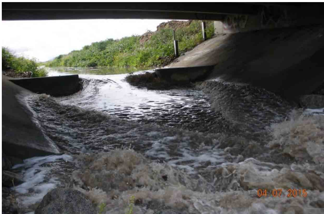
Figure 7-3. Field images of flow through the San Jon Road weir at flow rates of (upper image) 30 cfs and (lower image) 65 cfs
