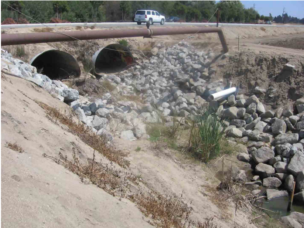
Figure 6-6: Image of the Laurel Road culverts, downstream end, on September 4, 2014.
