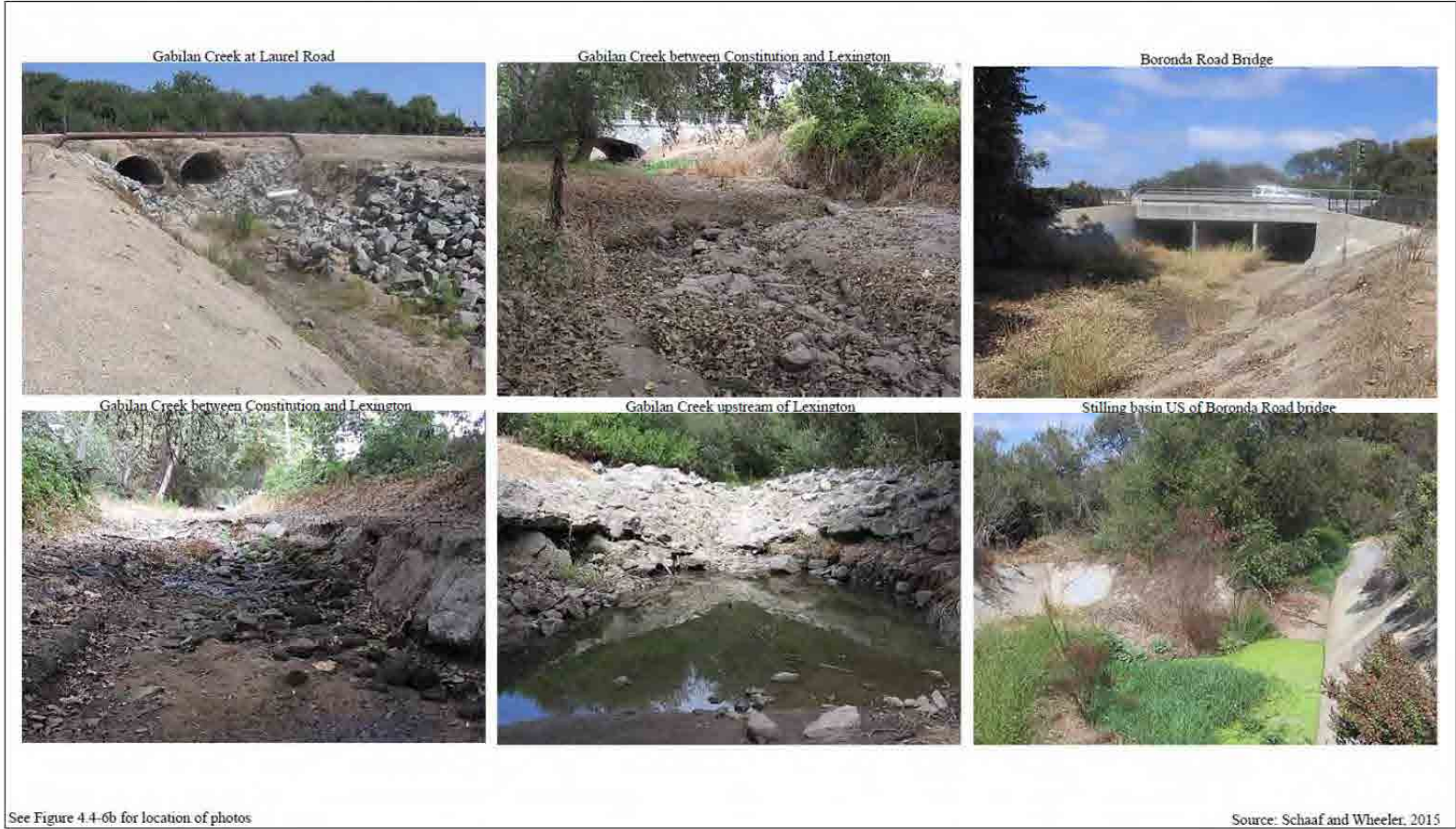
Figure 6-5. Photos of passage barriers downstream of Gabilan Creek.
