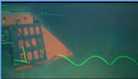
Deploying the cable to the MARS node
