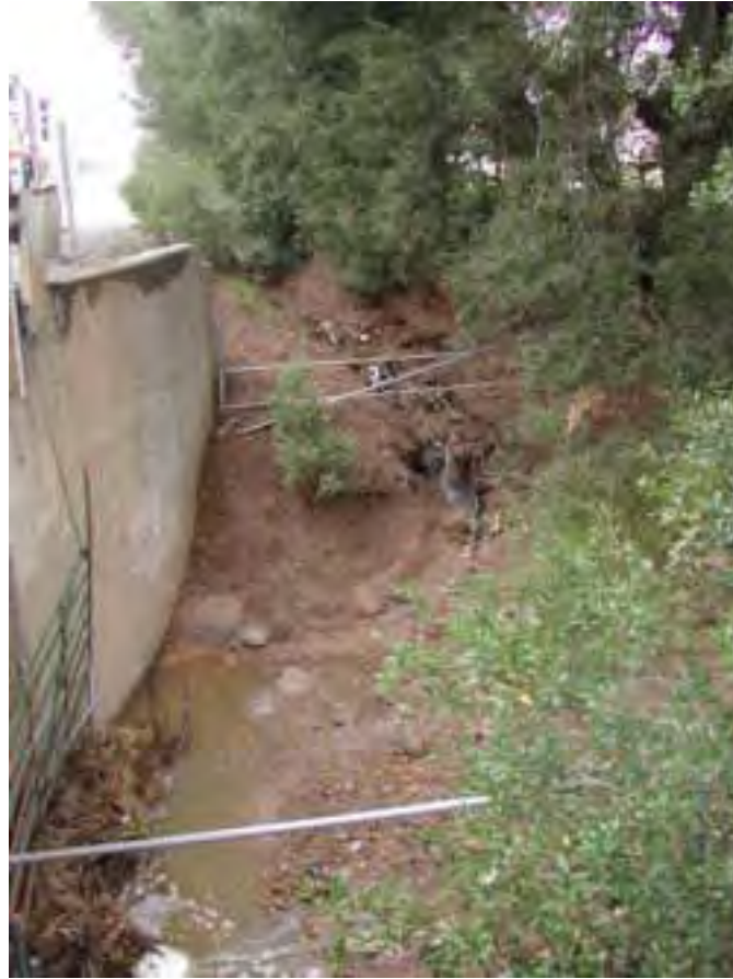
Figure 4.26. A road ditch on New Avenue entering Church Creek.
