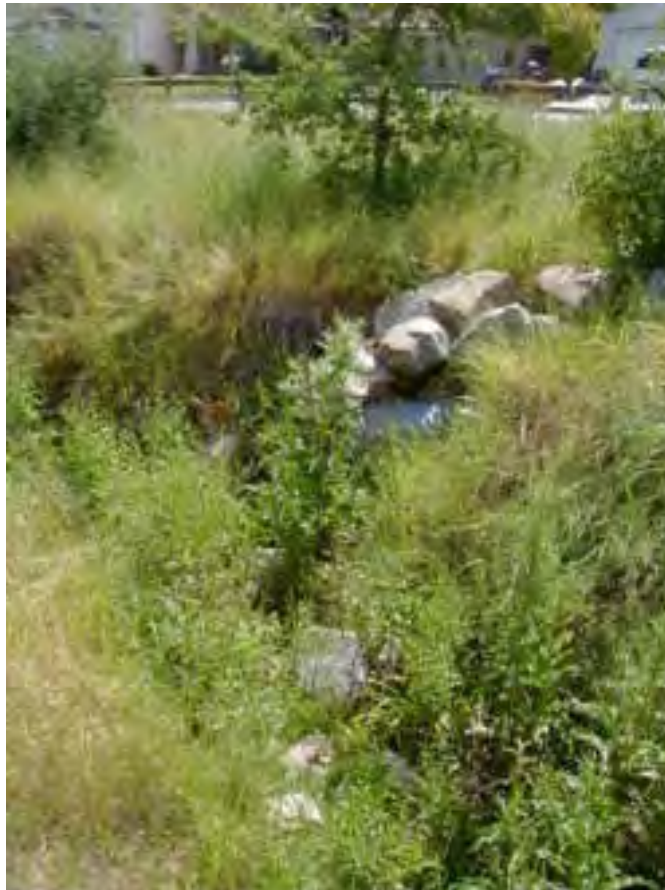
Figure 4.57. Babbs Creek in the Babbs Creek Park Preserve where young oak trees have been planted on the channel banks and riprap has been placed downstream of stormwater outfalls.
