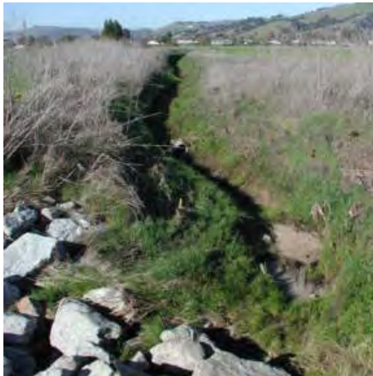
Figure 4.15. Tennant Creek upstream of Barrett Avenue.
