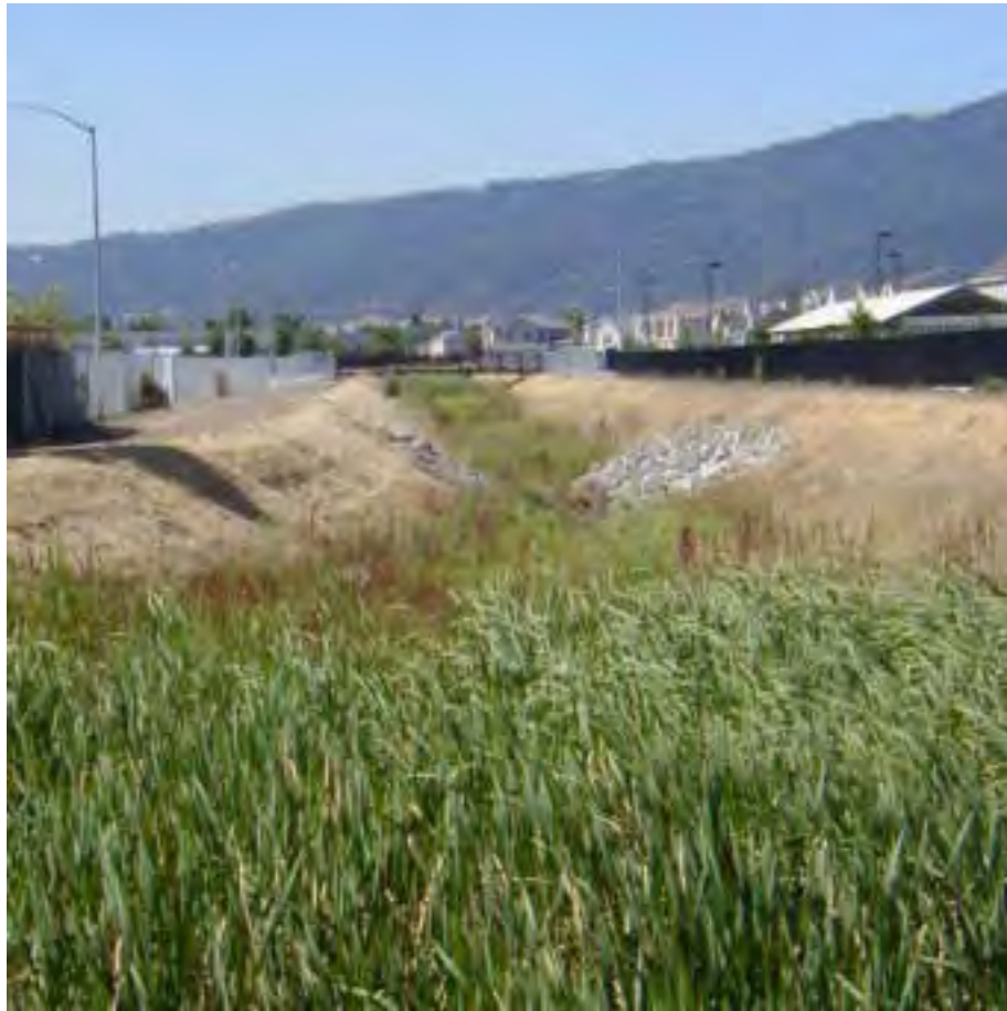
Figure 4.34. South Morey Channel upstream of the confluence with Lions Creek.
