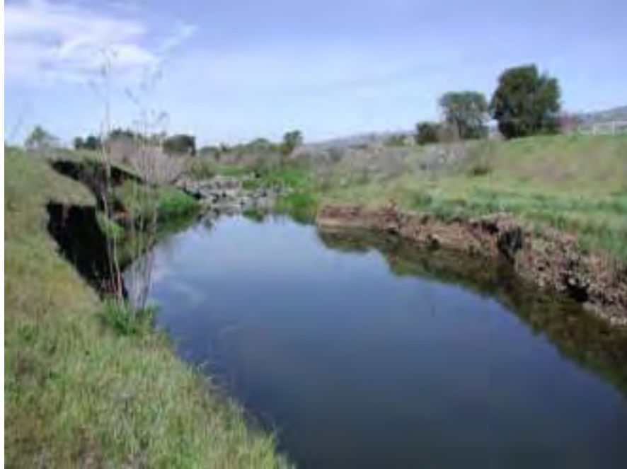
Figure 4.13. Bank and channel erosion on East Little Llagas Creek downstream of the confluence with Corralitos Creek.
