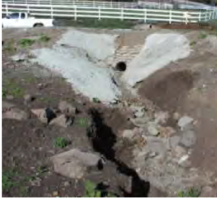
Figure 5.16. Examples of Drainage Culverts in Rural Residential Areas.
