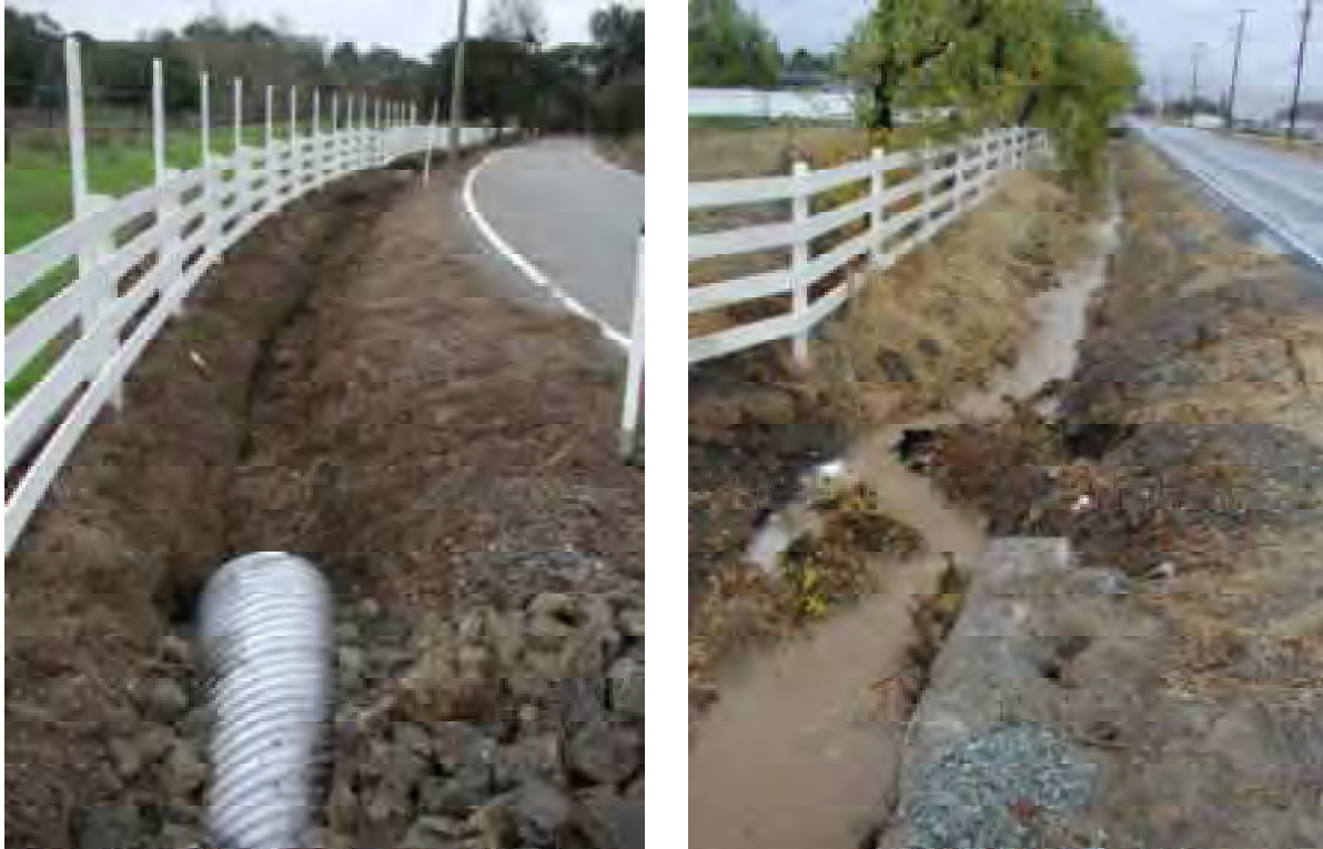
Figure 5.15. Examples of Road Ditches in Rural Residential Areas.
