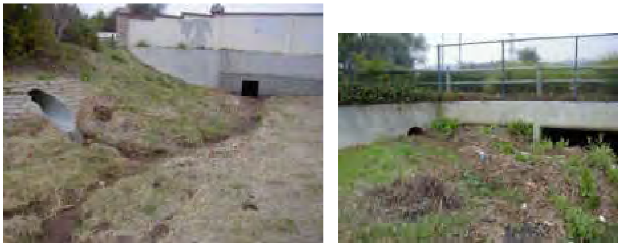
Figure 5.13. Example of Urban Drains and Flood Control Channel Hydromodifications.
