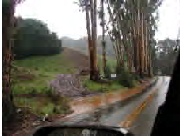
Figure 5.10. Example of Runoff from a Non-Surfaced Rangeland Road.
