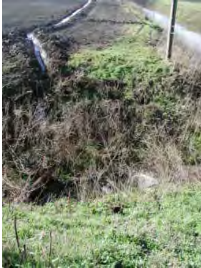
Figure 4.46. Water draining into Millers Canal via tail and stormwater drains.
