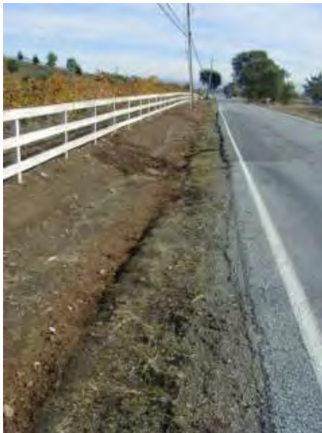
Figure 4.32. Day Creek road ditch on Day Road.
