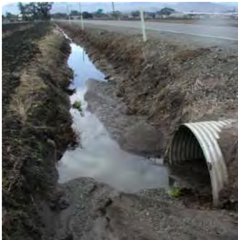
Figure 4.17. The Maple Creek road ditch on Maple Avenue.
