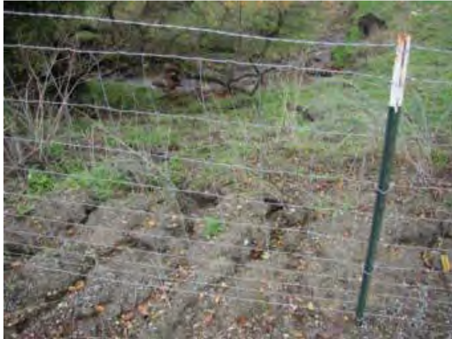
Figure 4.37. Location where runoff from Roop Road enters Live Oak Creek.
