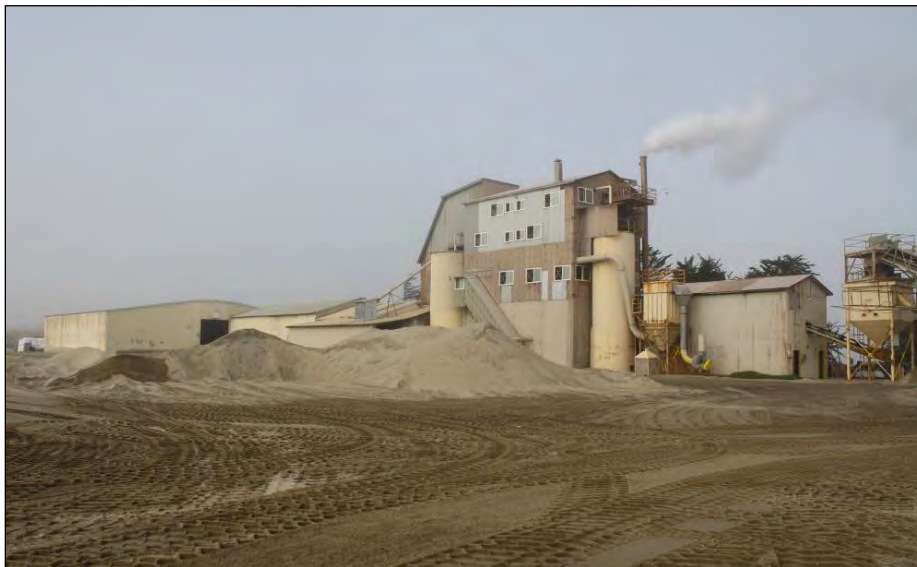
Figure 6. Overview of the Sorting Plant; view to the northwest.
