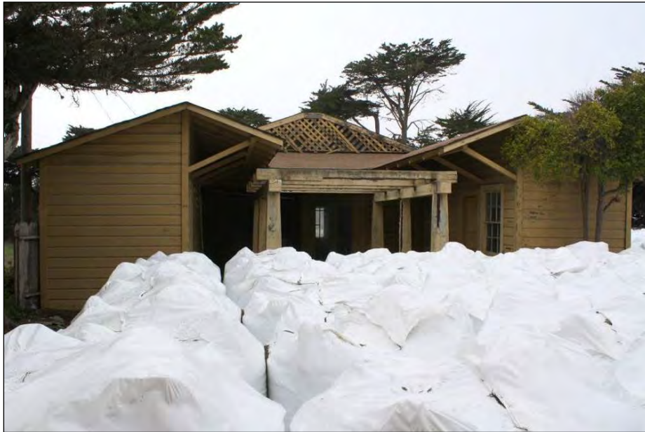
Figure 12. Overview of the Bunkhouse; view to the west.
