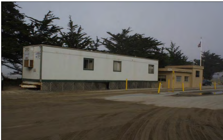
Figure 15. View of Scale House in background with adjacent office in foreground; view to the northeast.
