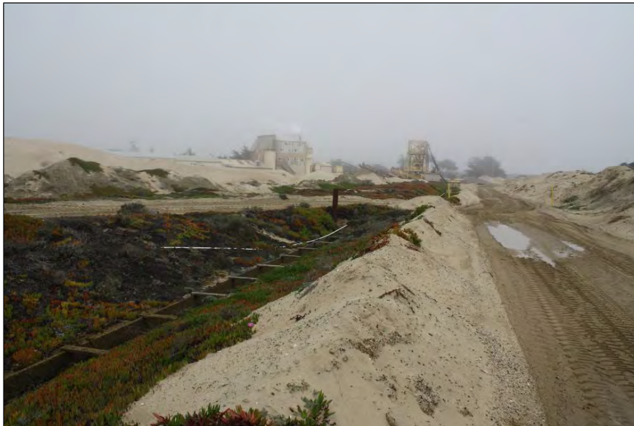
Figure 4. Overview of the project area, looking east.
