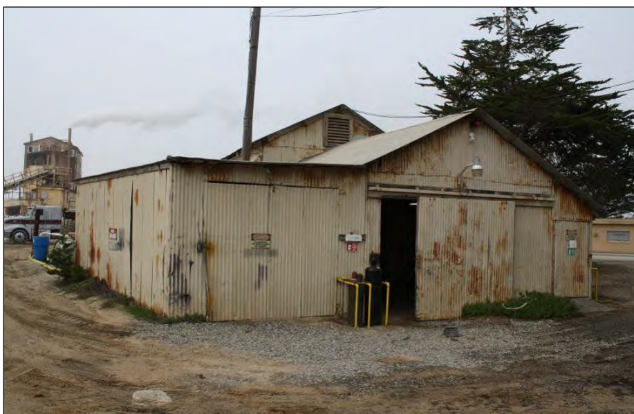
Figure 14. Overview of the Maintenance Shop; view to the northwest.
