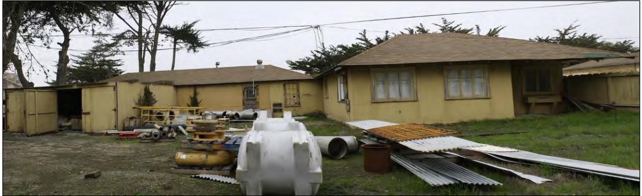
Figure 13. Overview of the Garage/Office; view to the north.
