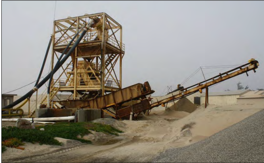
Figure 7. Overview of the Washing Plant; view to the northwest.
