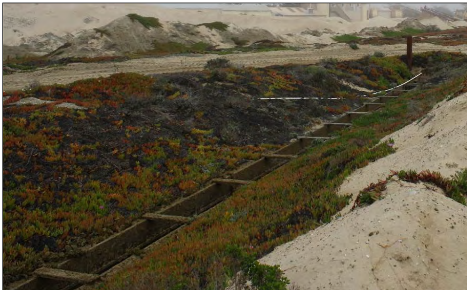
Figure 8. Overview of the Canal Flume; view to the northeast.
