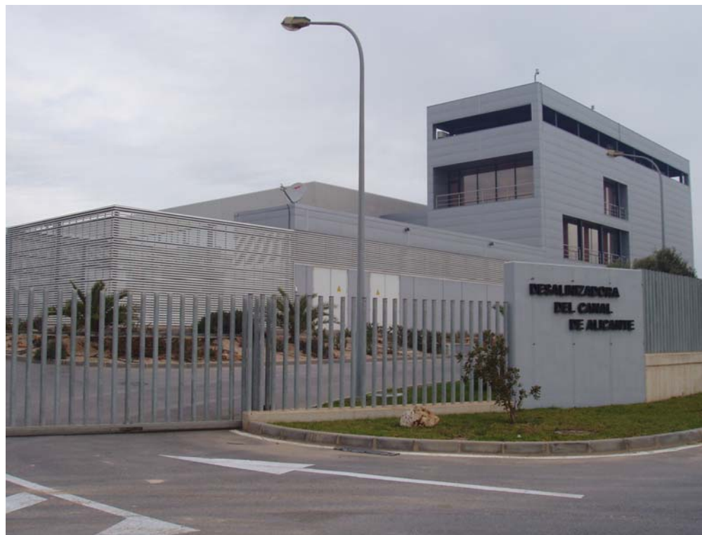
Desalination plant in Alicante/ WWF Spain
