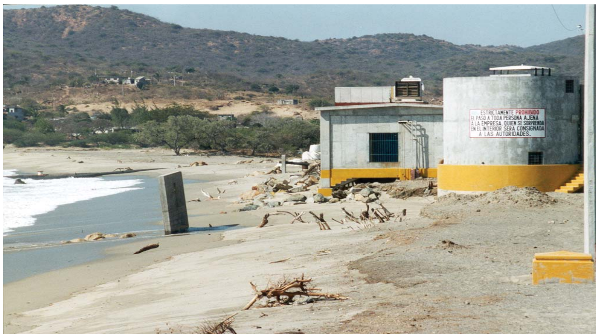
Figure 6 – Desalination Plant Intake Beach Well Erosion
