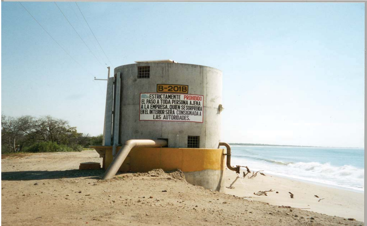
Figure 7 – 3.8 MGD Intake Beach Well of Large Seawater Desalination Plant
