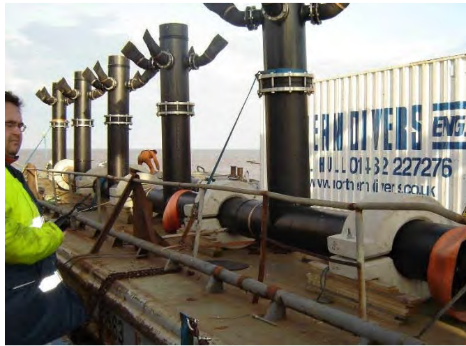
Figure 23. A brine diffuser with multiport rosettes.
