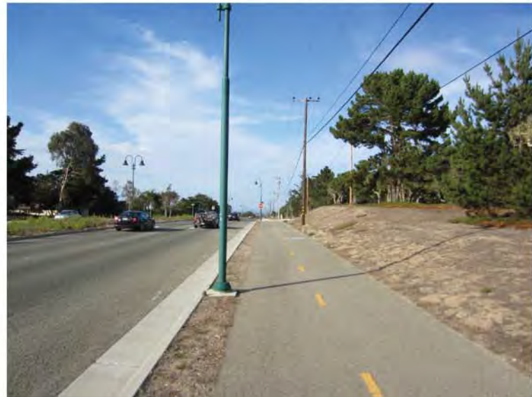
Photo 4. Northeast-facing view along General Jim Moore Boulevard of the proposed ASR injection/extraction wells site (ESA, 2013).
