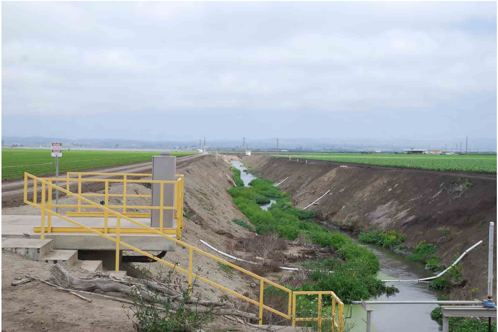
Figure 1. Blanco Drain at diversion site looking northeast towards Nashua Road
