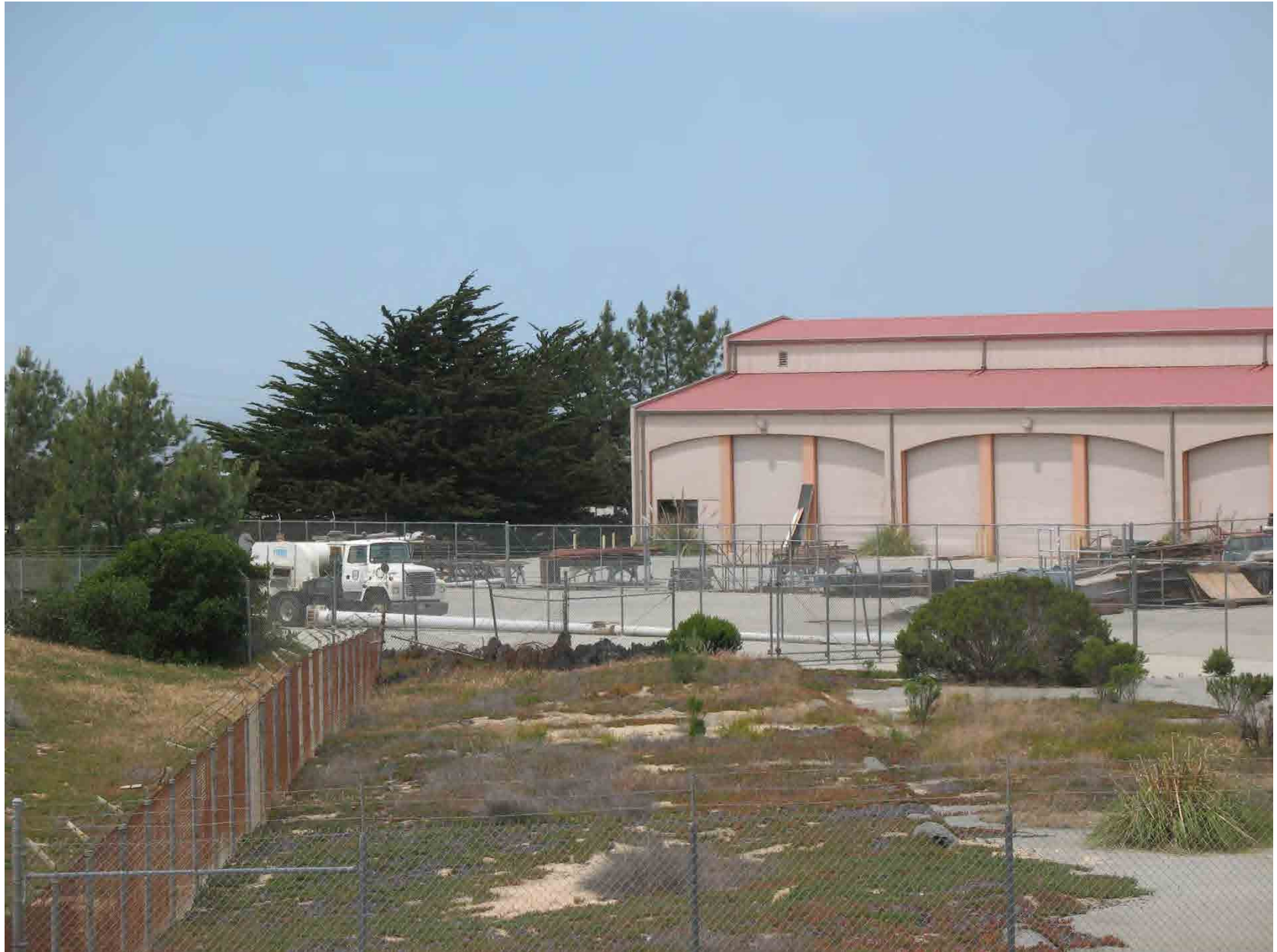
Figure 5. Booster Pump Station Site from Inter-Garrison Road looking north
