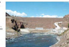
Iron Gate Dam, Klamath River
