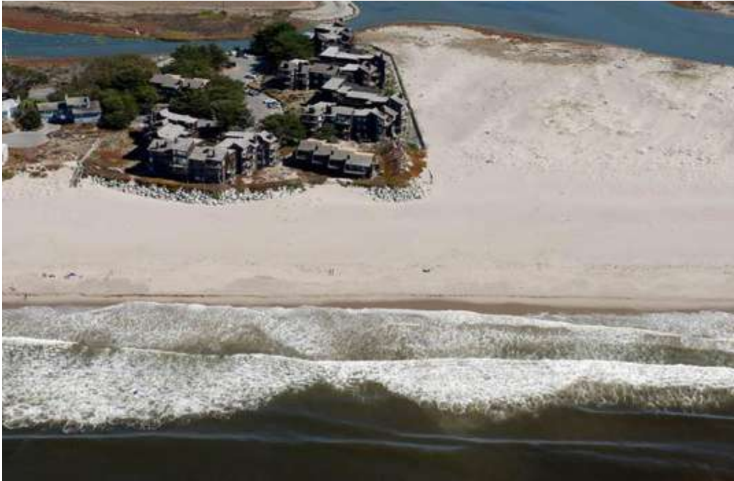
Figure 3-8. Aerial photograph of the southern end of the Pajaro Dunes-Sunset State Beach BECA, dated October 2013. The extensive development on active sand dunes is subject to wave attack and inundation from the adjacent mouth of the Pajaro River. Source: Adelman and Adelman
