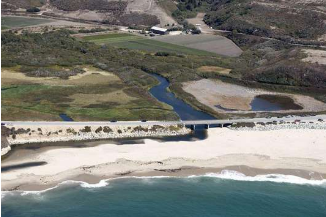
Figure 3-10. Aerial photograph of the Scott Creek Beach BECA and sediment impaired Scott Creek Lagoon, dated Sep 2010. The bridge and raised roadway constrict the mouth of Scott Creek and effectively isolate the lagoon from the open coast. Source: Adelman and Adelman.
