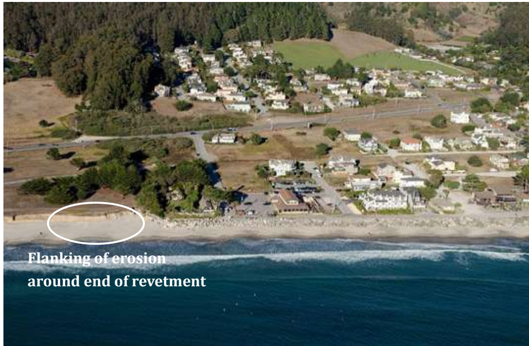
Figure 3-5. Aerial photograph of the southern section of the El Granada County Beach BECA, dated September 2013. Erosion is flanking the north end of the rock revetment fronting Mirada Road. Source: Adelman and Adelman
