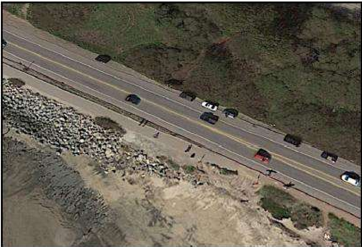
Figure 7-2. Vulnerable section of Highway 1 at Surfer’s Beach
