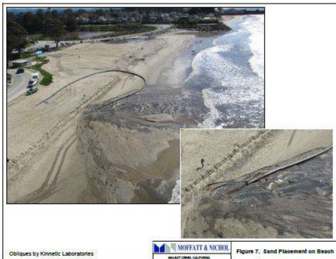
Figure 4-3. Beach nourishment operations at Twin Lakes State Beach. Source: Moffatt & Nichol et al., (2011)
