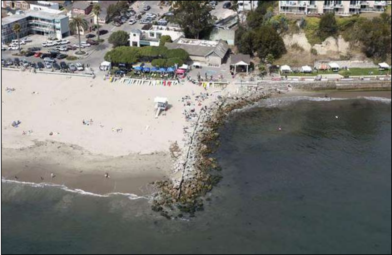
Figure 4-8. Aerial view of rubblemound groin at Capitola. Source: Adelman and Adelman (2010)
