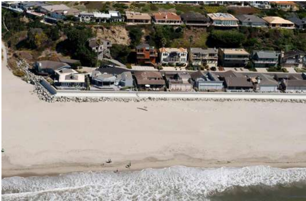
Figure 3-6. Aerial photograph of the Rio Del Mar-Via Gaviota BECA, dated October 2013. The extensive development on the back beach is largely protected from wave attack and inundation by a seawall and rock revetment. Source: Adelman and Adelman
