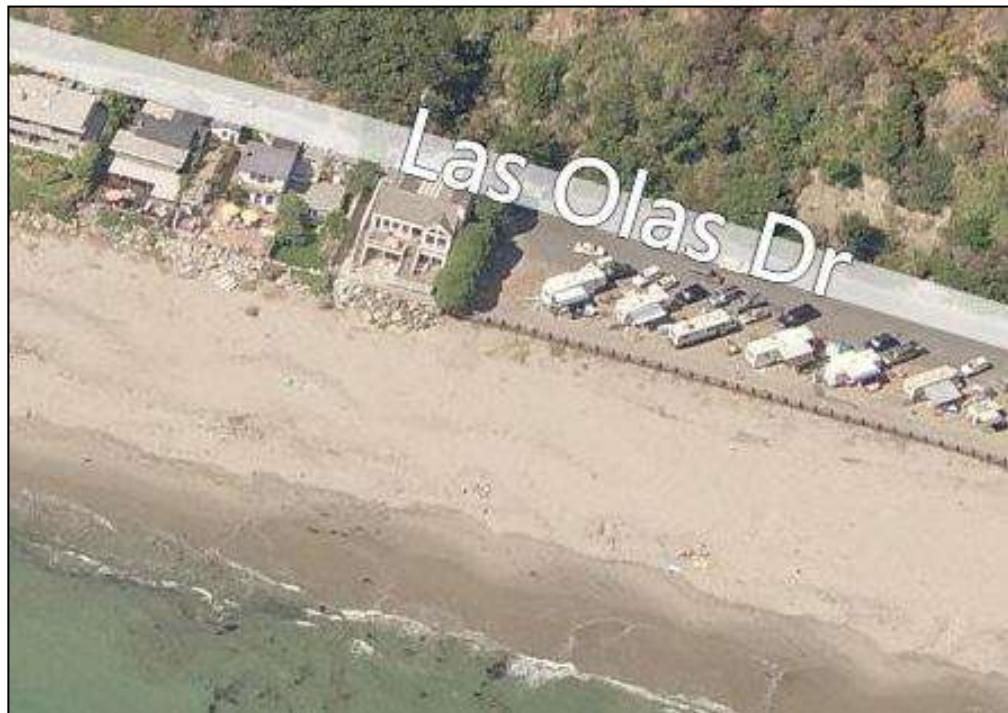
Figure 7-16. Armoring at Seacliff State Beach. Source: Bing Maps
